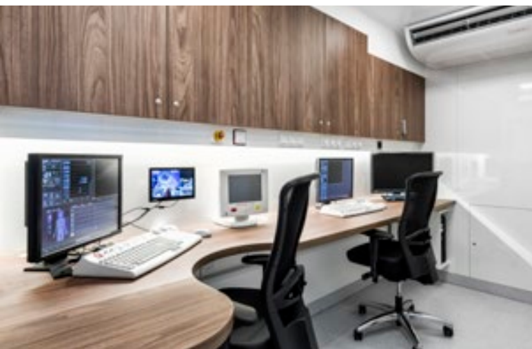
Control room in the Mobile Trailer.
