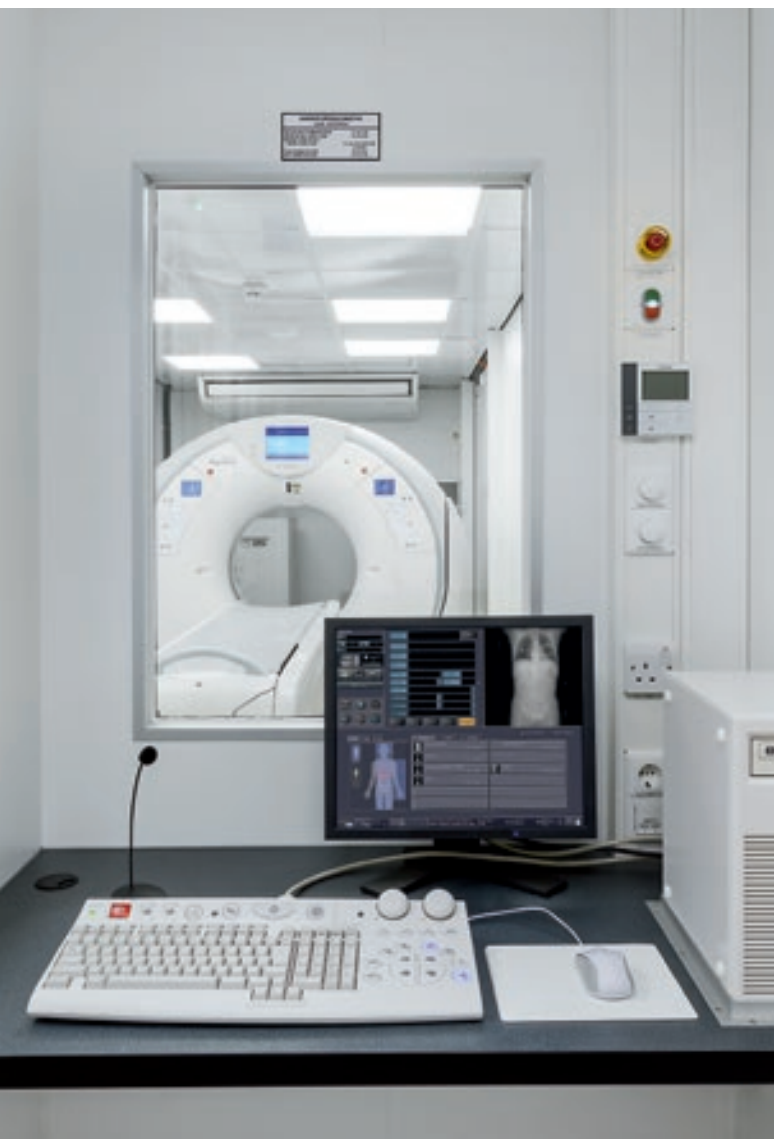
Control room of the CT Scan Units.
